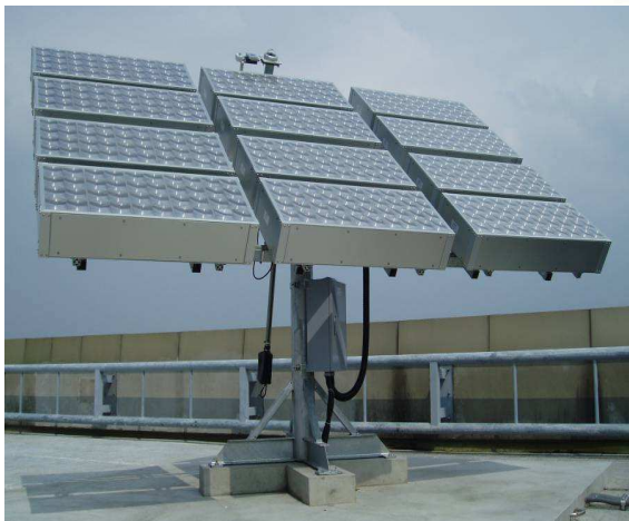
1.5kW Roof-top HCPV – Spirox, Hsin-Chu, Taiwan
